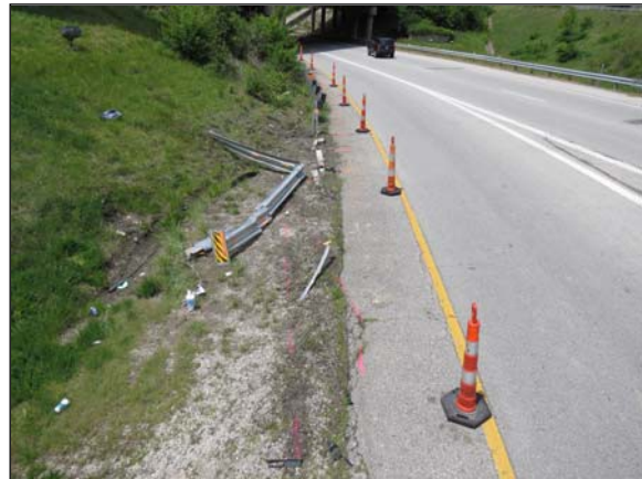
Figure 1: Overview of crash scene with X-Lite guardrail end treatment (detached)
