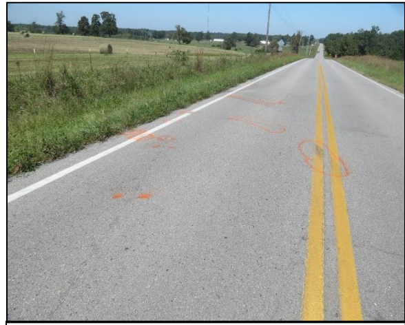
Figure 6: View northeast to area of impact in the southbound lane
