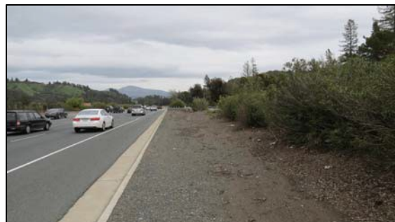
Figure 3. Roadway departure, looking east
