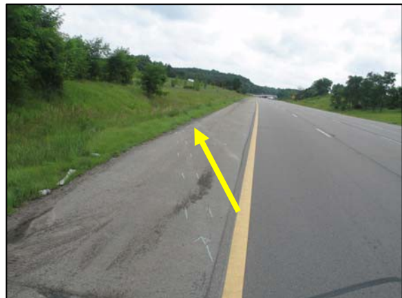
Figure 2: Northeast roadway departure
