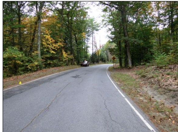
Figure 2: West-facing trajectory view of the roadway in the vicinity of the crash.
