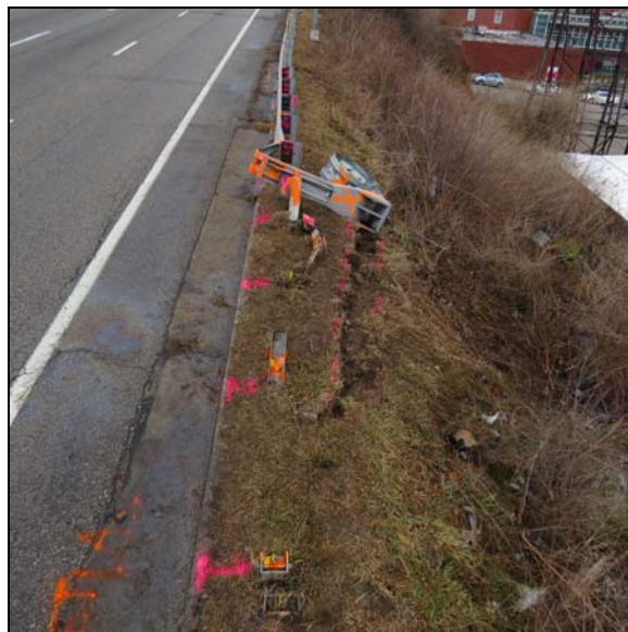
Figure 1: SKT end treatment and guardrail
