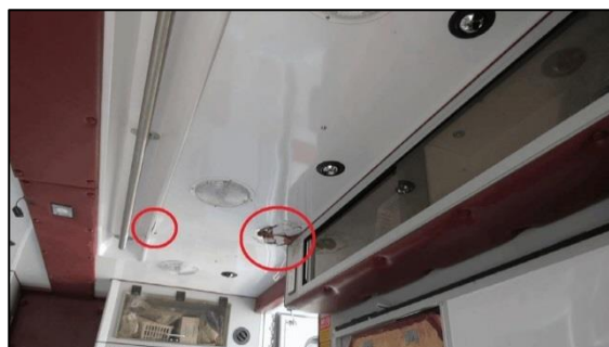
Figure 9. Patient compartment damage, 2004 Ford E-350 ambulance.
