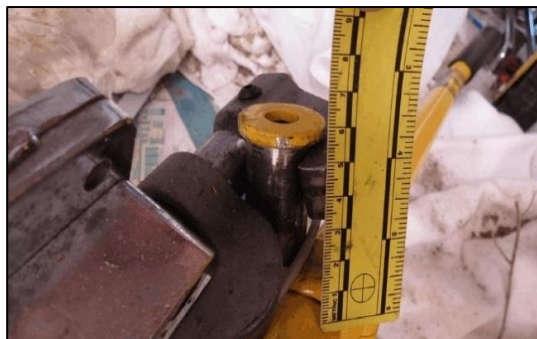
Figure 13. Lower frame rail/pin.
