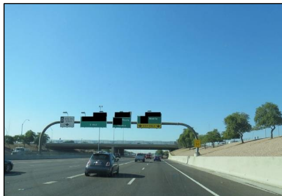
Figure 2. Westbound traffic lanes.
