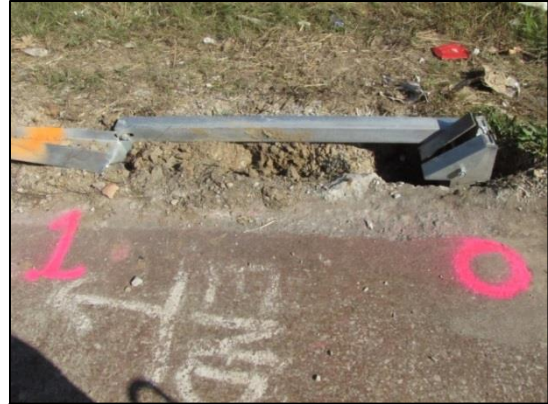
Figure 9. East-facing image depicting Post 0, Post 1, and the ground strut.
