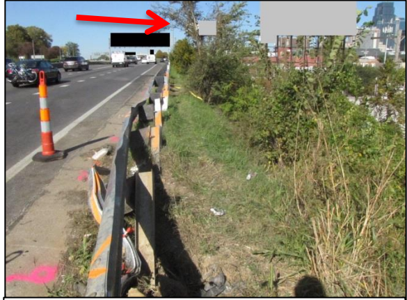
Figure 6. North-facing view depicting the vehicle's path along the field side of the guardrail. The red arrow referenced the small diameter tree contacted by the Ford.
