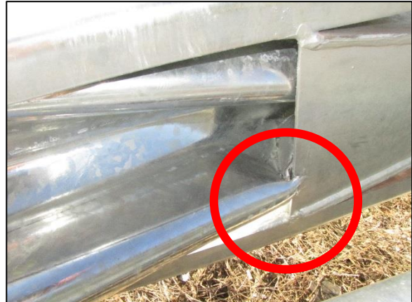
Figure 11. Close-up west-facing view of the restricted W-beam in the end terminal.
