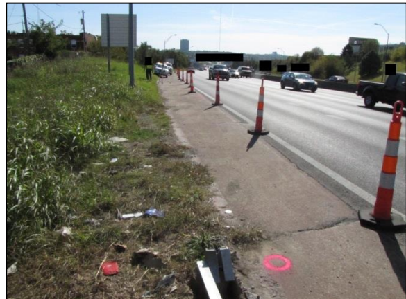
Figure 3. South-facing look back view for the point of impact depicting the roadway curvature.
