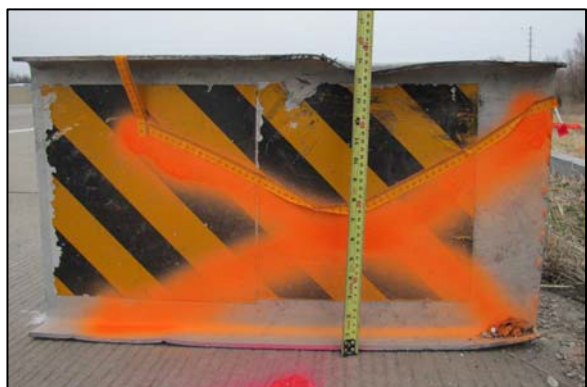
Figure 5. The damaged end terminal.
