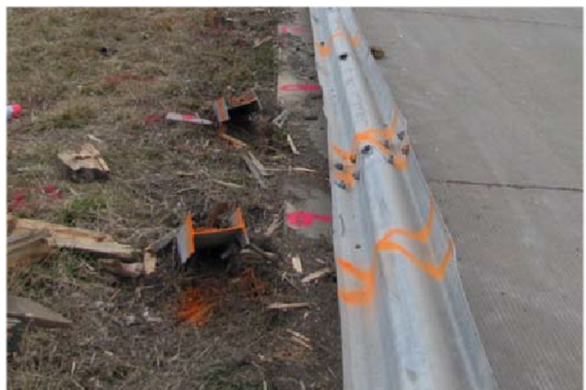
Figure 10. Bent posts 8 and 9, view west.
