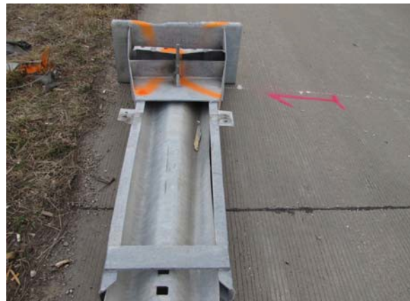
Figure 7. The field side of the end terminal.
