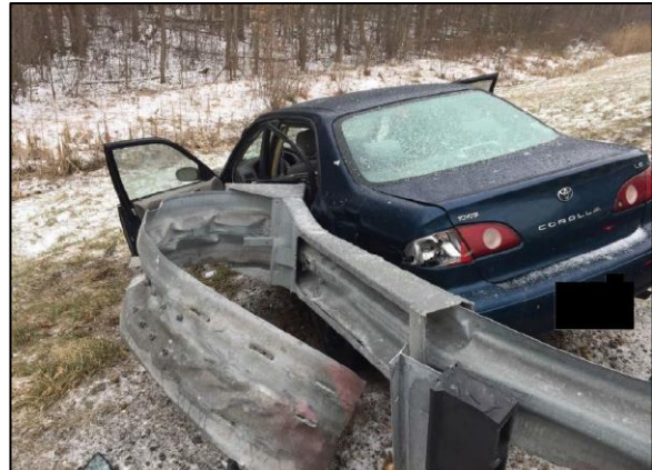
Figure 6. Southwesterly view of the final rest position of the Toyota engaged against the terminal end. Image provided by the PTC.
