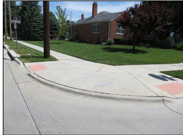
Figure 6: Volkswagen’s northeast approach to curb impact and final rest near house; final rest of the Chevrolet against the utility pole in the foreground
