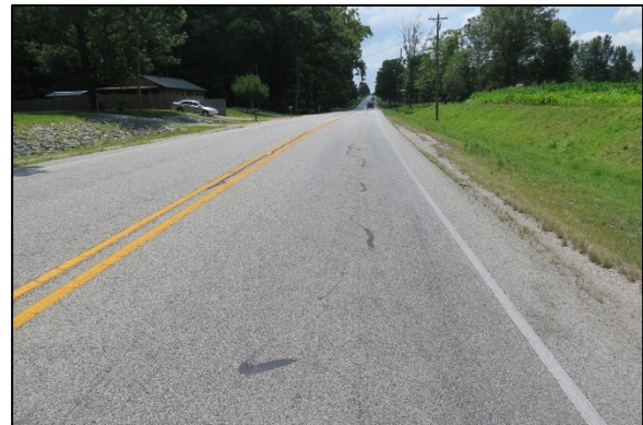
Figure 2: Southbound approach of the Honda.
