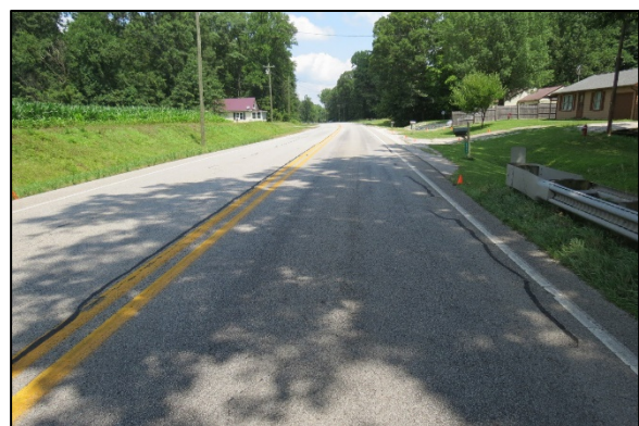
Figure 3: Northbound approach of the Ford.
