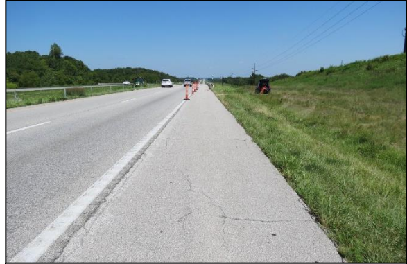
Figure 3. Northbound approach of the Nissan to the end terminal.
