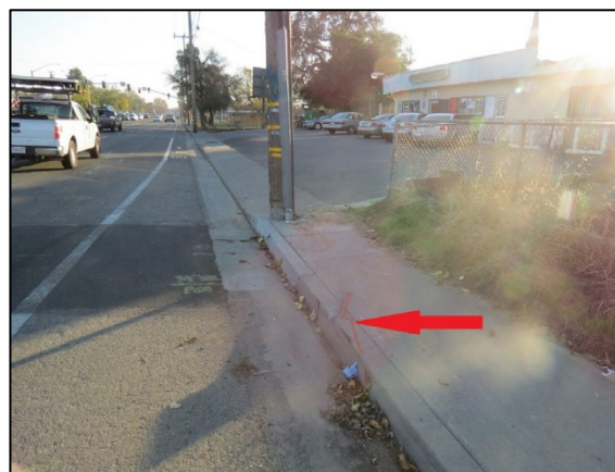
Figure 3. Struck curb, looking south.
