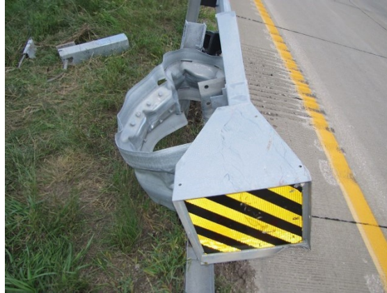
Figure 5. SKT guardrail, left shoulder looking east
