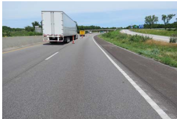
Figure 2. Northbound view of the roadway.
