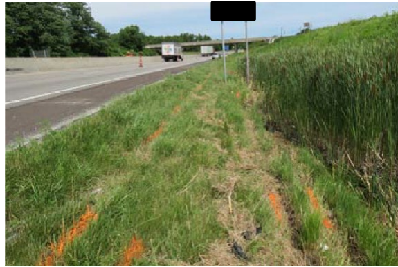
Figure 3. North approach to the sign posts impacts.
