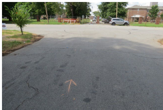
Figure 3. North view, start of tire mark and approach to the intersection
