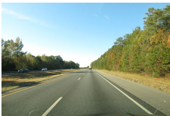
Figure 3. Southbound view of the roadway for the Peterbilt's and Nissan's pre-crash travel
