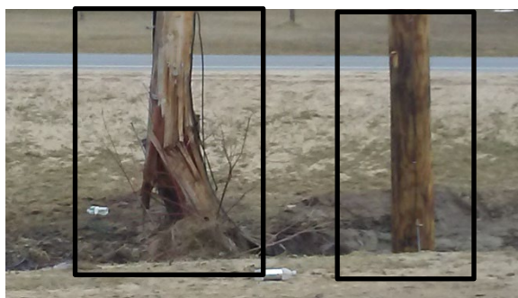
Figure 3. North-facing view at the crash site of the struck and fractured utility pole (left) and the replaced utility pole (right). Image supplied by the owner of the Chevrolet.
