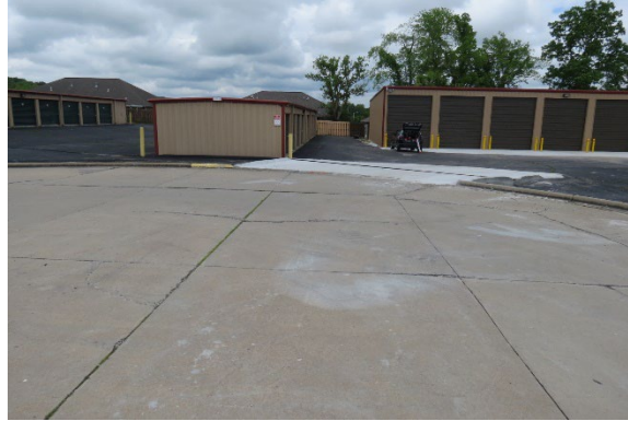
Figure 3. North view, entrance into the storage facility
