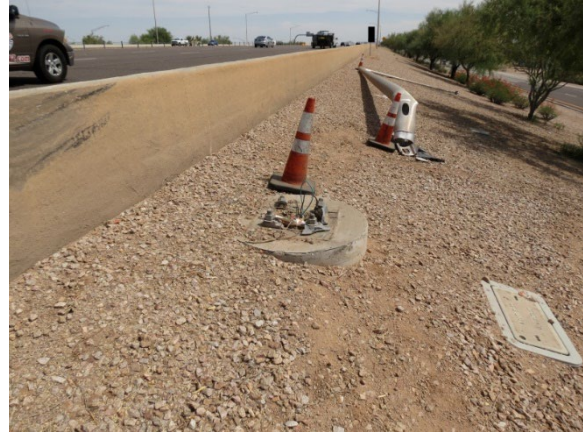
Figure 6. POI Event 2, light pole looking south
