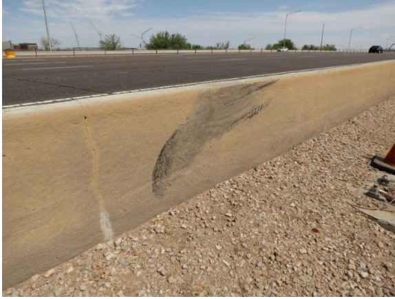
Figure 5. POI Event 1, retaining wall looking south
