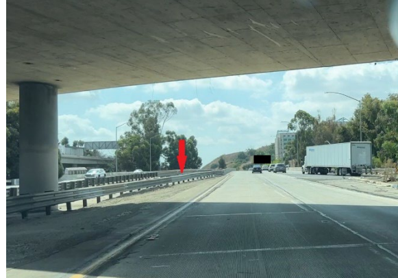
Figure 6. Event 2 (guardrail), Event 3 (rollover), Event 4 (guardrail, looking south)
