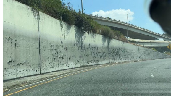
Figure 4. Ramp transition to southbound roadway, looking southeast
