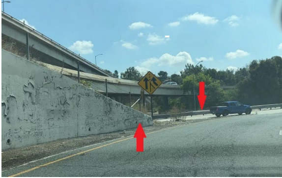
Figure 5. Event 1 (wall), Event 2 (guardrail, looking southeast)
