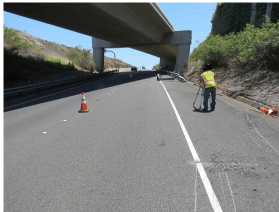
Figure 3. Crash site looking north to guardrail end terminal
