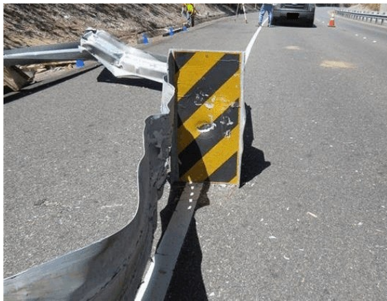
Figure 4. ET-Plus impact head end terminal
