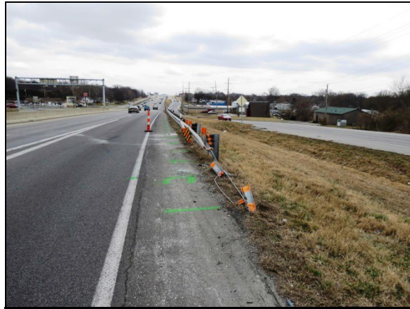
Figure 3: East-facing view of the crash site and the X-Lite guardrail.
