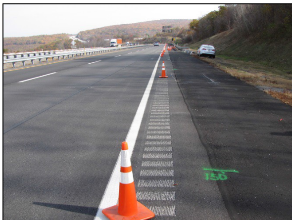
Figure 2: East-looking view of the crash site 93 m (150 ft) from post 1.
