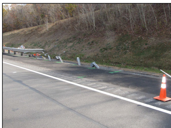
Figure 3: Southeast-looking oblique view of the crash site.
