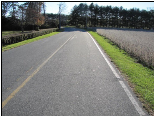
Figure 2: South-facing view of the roadway for the RAM's pre-crash travel trajectory.
