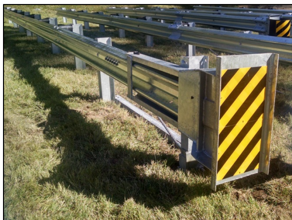
Figure 6: Image depicting an exemplar ET-Plus end terminal installation.
