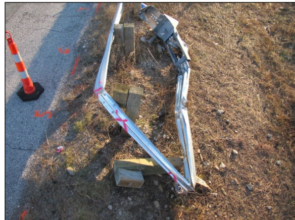
Figure 1: The damaged guardrail and ET-2000
