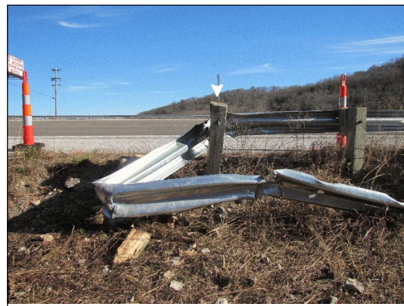
Figure 10: Slightly displaced post 5, view east
