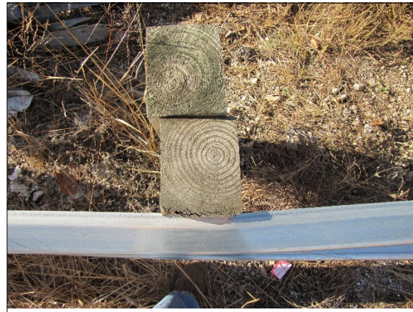
Figure 11: Block-out of post 6 slightly damaged
