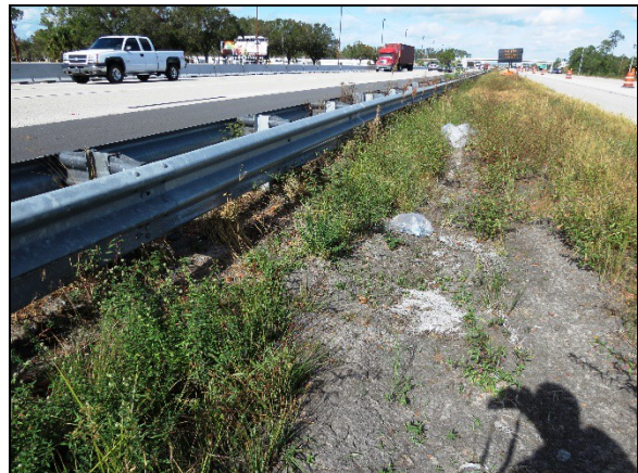
Figure 4: Northwest-facing view of the guardrail barrier system, replaced following the crash.
