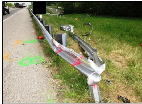
**Figure 10: East-looking image of the deformed W-beam wrapped around Post 7.**
