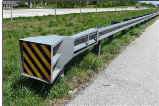
**Figure 7:** East-looking image depicting an exemplar SKT guardrail end treatment located on the left side of the interstate highway across from the crash site.
