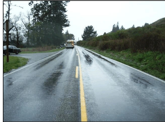
Figure 2. Crash site looking west (police photo)
