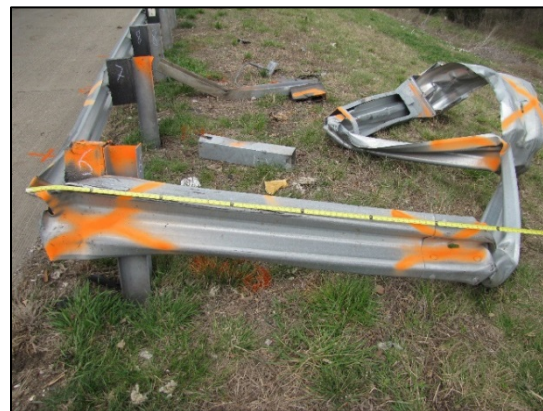
Figure 11: Four kinks in the guardrail and extruded guardrail from the end terminal, each black mark on tape is 0.3 m (1.0 ft), view west
