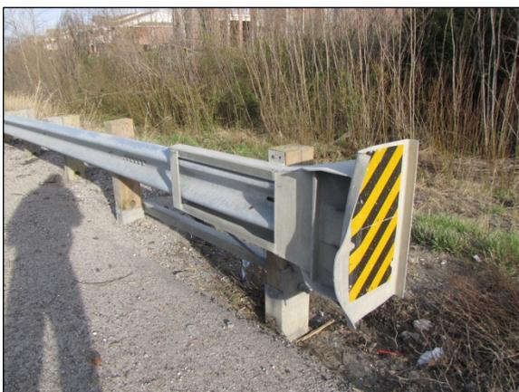
**Figure 4:** Image depicting an exemplar ET-Plus installation located near the crash site.
