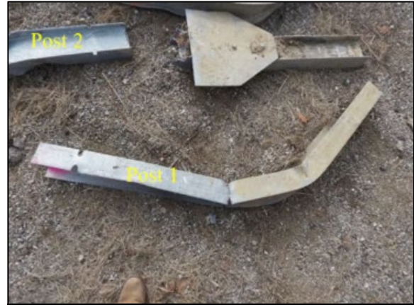
Figure 8: Damaged posts 1 and 2
