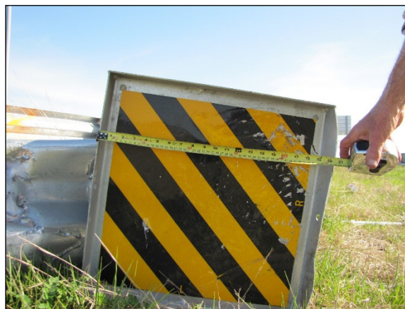
Figure 6: The damaged SKT
