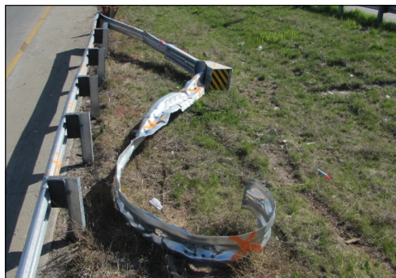
Figure 7: Extruded guardrail from the SKT and posts 6 to 12, view south
