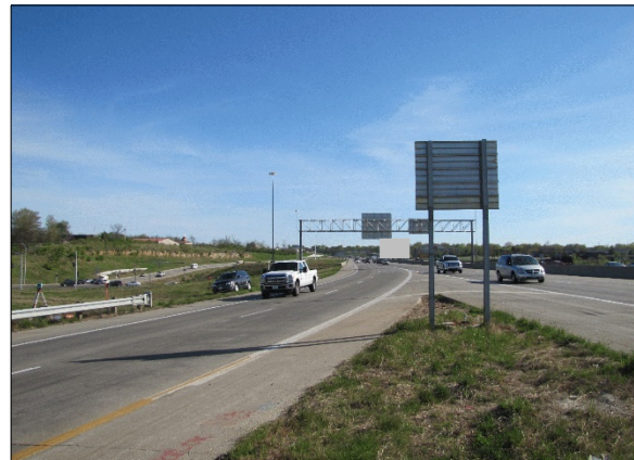
Figure 3: View south from the end of the damaged guardrail to the approach of the Kia
