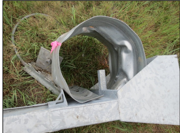
Figure 7: Extruded section of guardrail to the field side of the SKT
