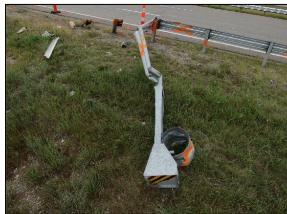
Figure 9: Kinks in the guardrail
