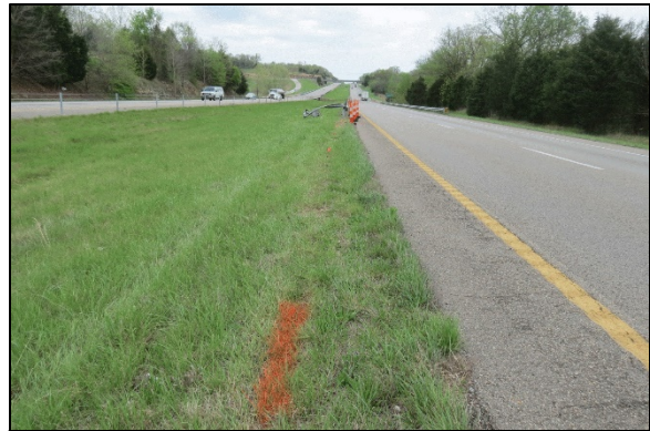
Figure 4: Approach of the Ford to impact with the End terminal, view northwest
