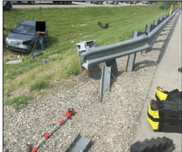
Figure 1: On-scene police image of the damaged end treatment and the final rest position of the Hyundai.
