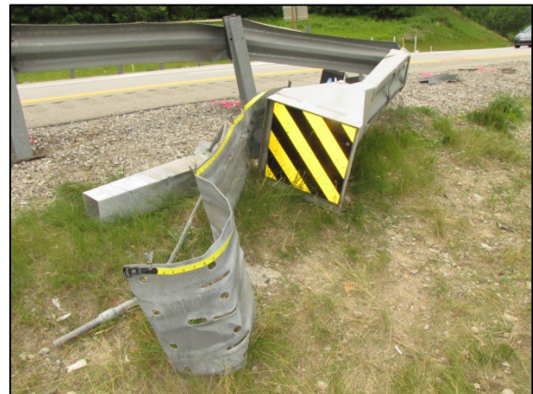
Figure 6: Southeast-facing image depicting the struck end terminal and the extruded W-beam.
