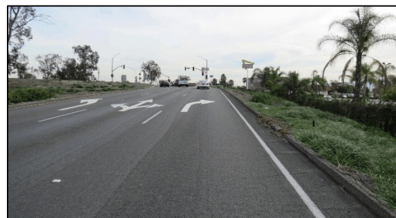
Figure 3. Eastbound approach along ramp.
