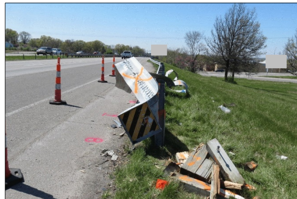
Figure 7: The damaged end terminal, extruded guardrail, and final rest location of the Chevrolet
