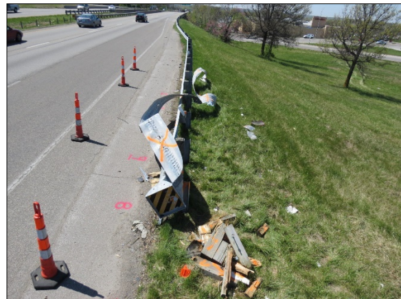
Figure 1: The damaged end terminal and guardrail, view west
