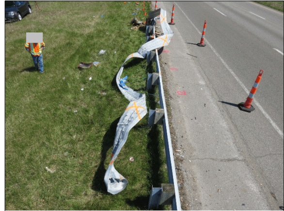
Figure 9: View upstream (east) to the extruded guardrail
