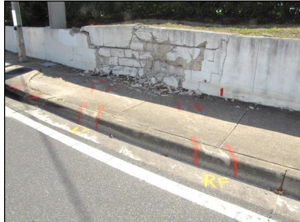
Figure 4: Image showing the Honda's impacts with the curb and concrete block wall.
