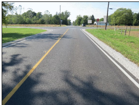
Figure 3: Westbound approach of the Dodge to the intersection.
