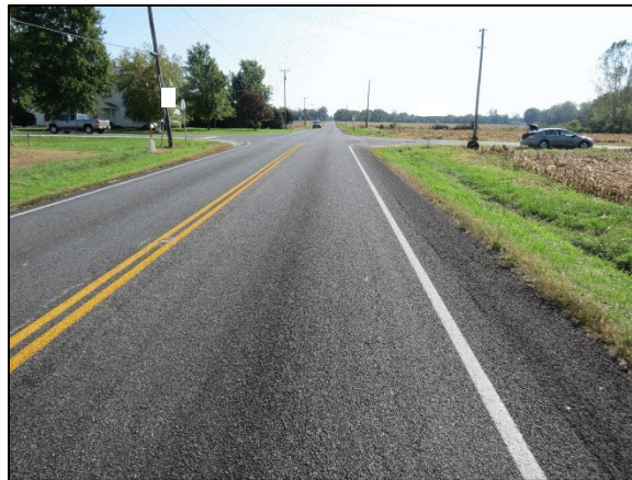
Figure 2: Southbound approach of the ambulance to the intersection.
