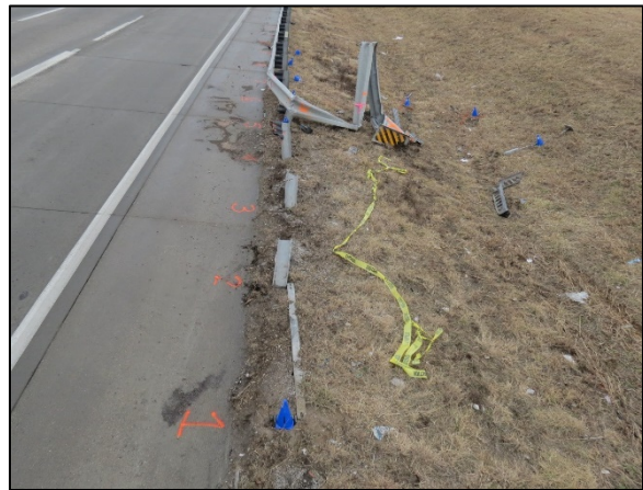
Figure 8: Damaged and displaced posts and guardrail, view southeast.
