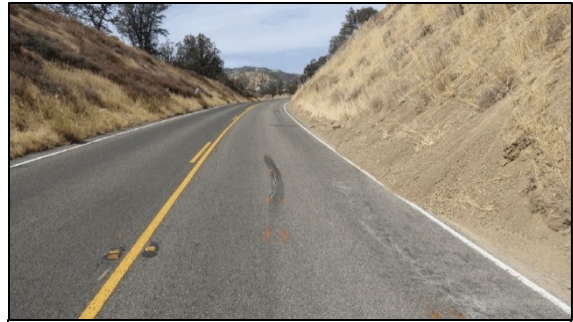
Figure 3. Area of embankment impact
