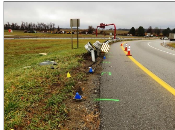
Figure 5: East-facing trajectory view of the Hyundai at the point of impact with the end treatment.
