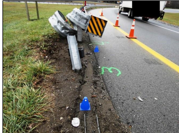
Figure 1: East-looking trajectory view of the Hyundai showing the struck guardrail end-treatment.
