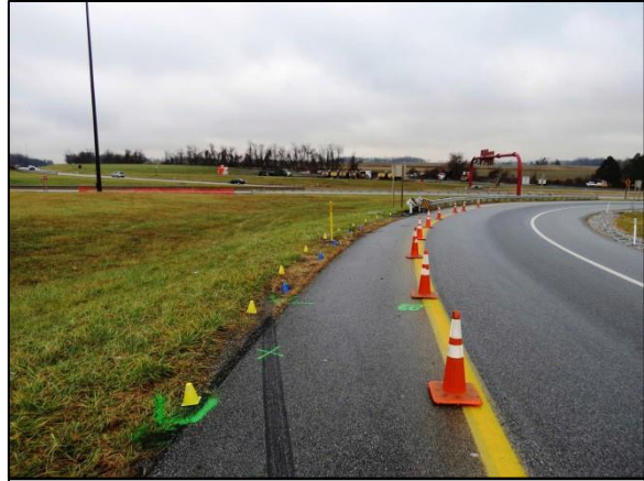
Figure 4: East-facing image showing the yaw marks along the Hyundai's trajectory.
