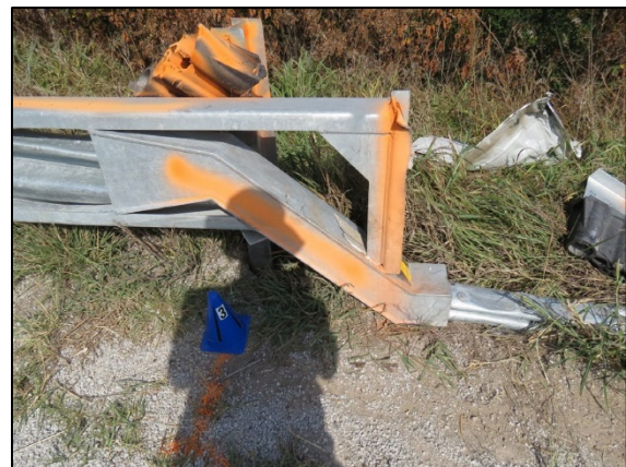
Figure 6. Trinity SoftStop guardrail end terminal, looking north
