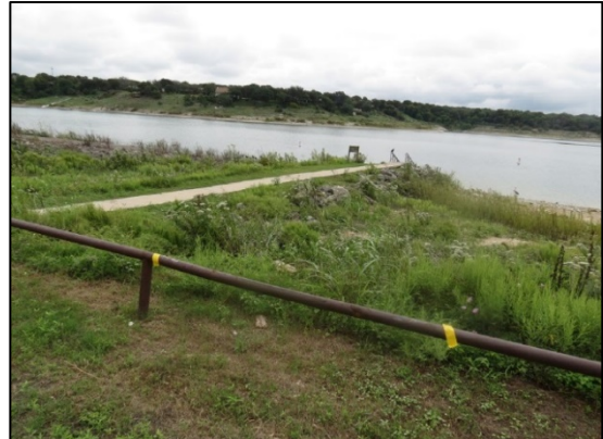
Figure 4. Impact with pipe rail, looking southeast.
