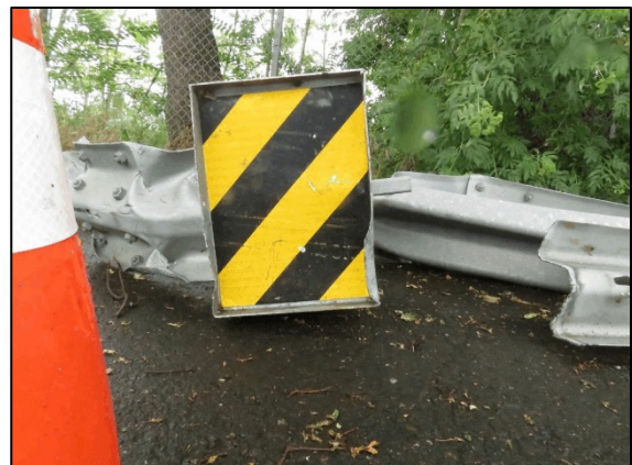
Figure 4. FLEAT end terminal impact face.
