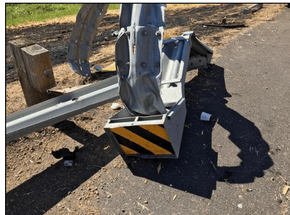
Figure 2. FLEAT guardrail end terminal struck by 2013 Toyota Avalon (Caltrans [California Department of Transportation] photo).
