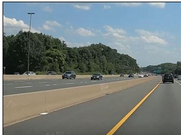
Figure 3: Southeast-facing view of the concrete barrier in the area of the crash.
